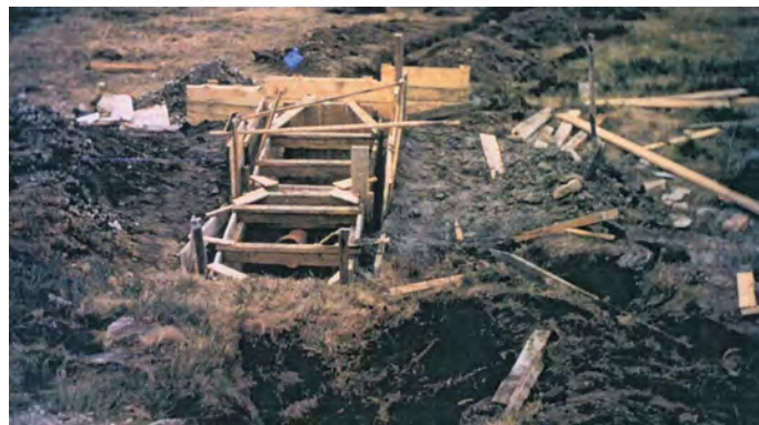
Septic Tank Construction (Photo by D. Pinkstone)
