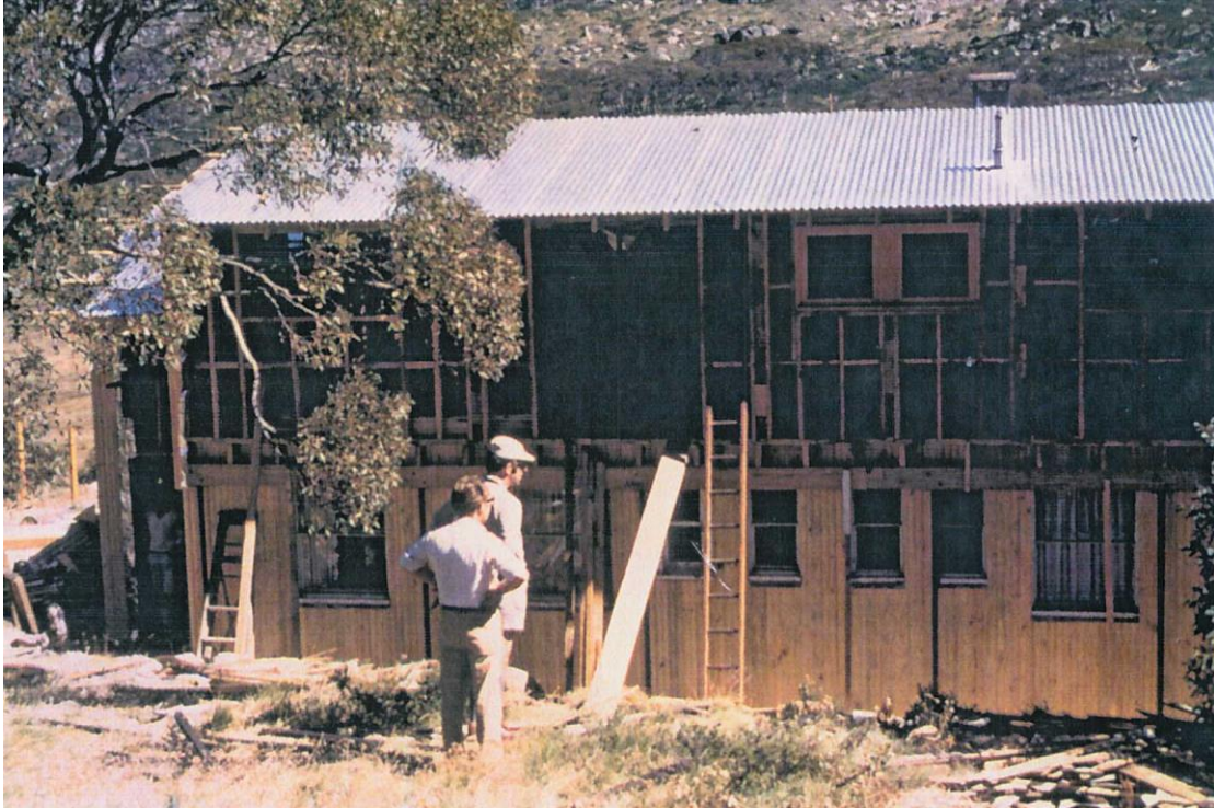
John Bible and George Failes inspecting progress (Photo by J. Brennan)
